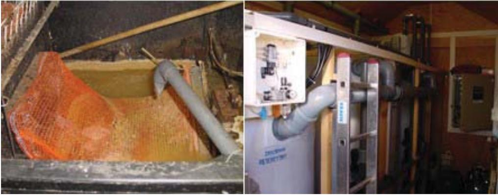
Fig. 2. Biovac® wastewater treatment plant at West Spitsbergen a) bag screen , b) retention tank [10]
