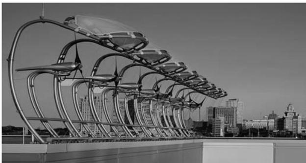
Ill. 3. Architectural Wind turbines by AeroVironment [5]
